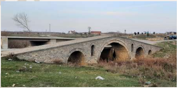
The bridge is over the Mirusha/Miruša river. It is characteristical arched bridge of the region from the XVIII and XIX centuries.
